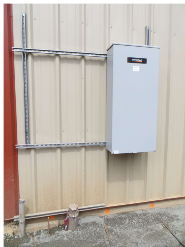
Electrical Transfer Switch connects to TPUD and Generator
