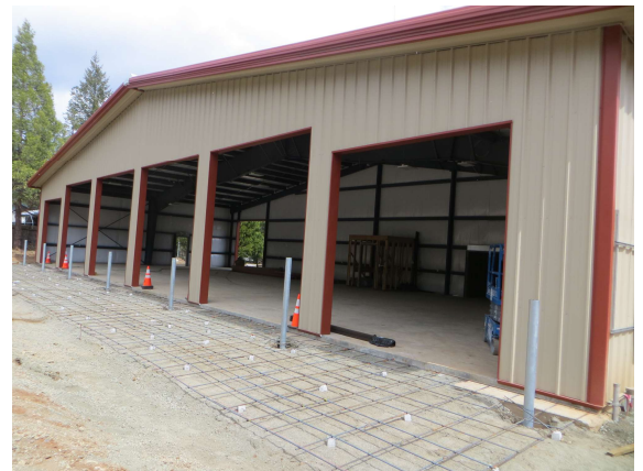
Rebar for concrete in front of building.
